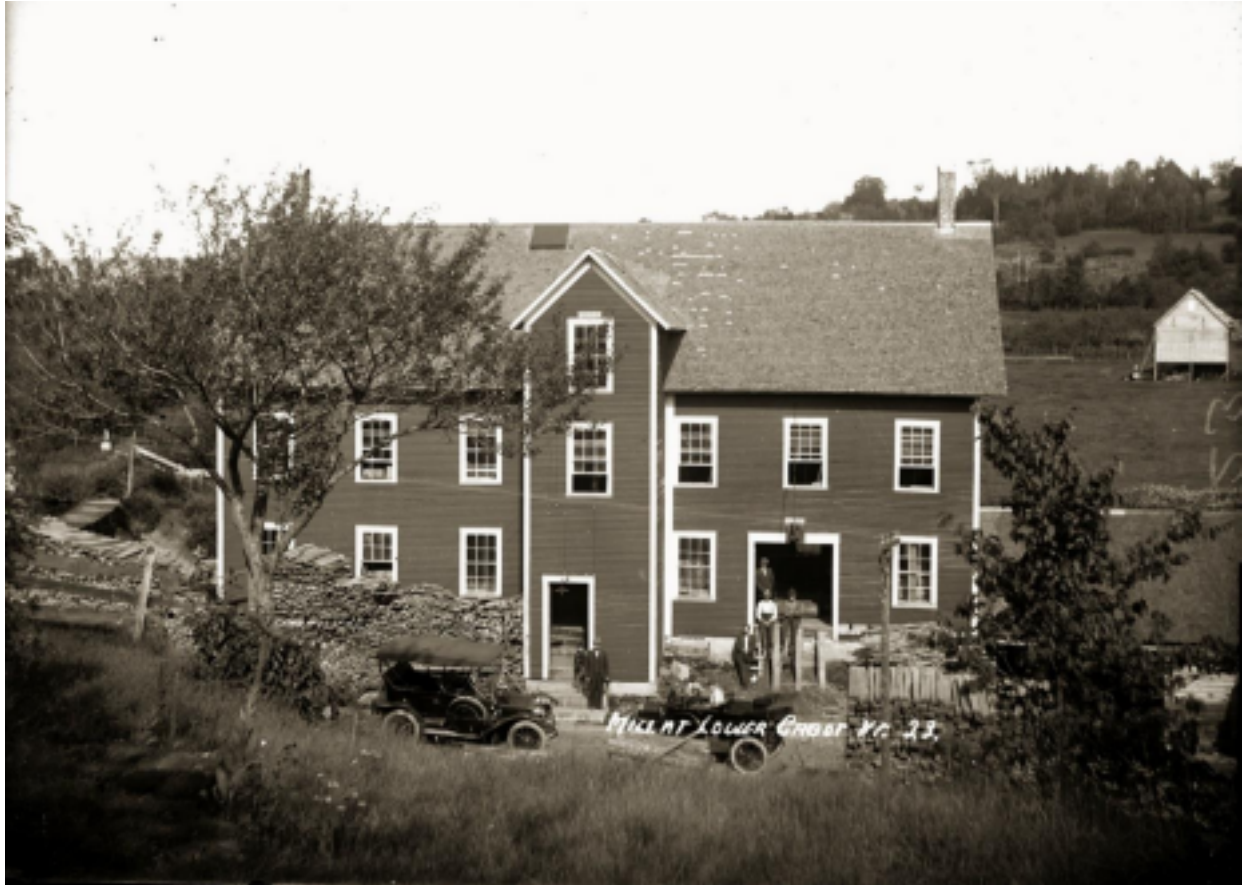
Figure 11. View east ca. 1910 – 1920 of mill at Lower Cabot, VT (Courtesy Penobscot Marine Museum, Eastern Collection, LB2007.1.10231). Note: dam at left behind woodpile (with no visible concrete and no water flowing over the spillway), electric lights and wiring on the building, type of vehicles in the image, and roof of structure to the right of the mill.
