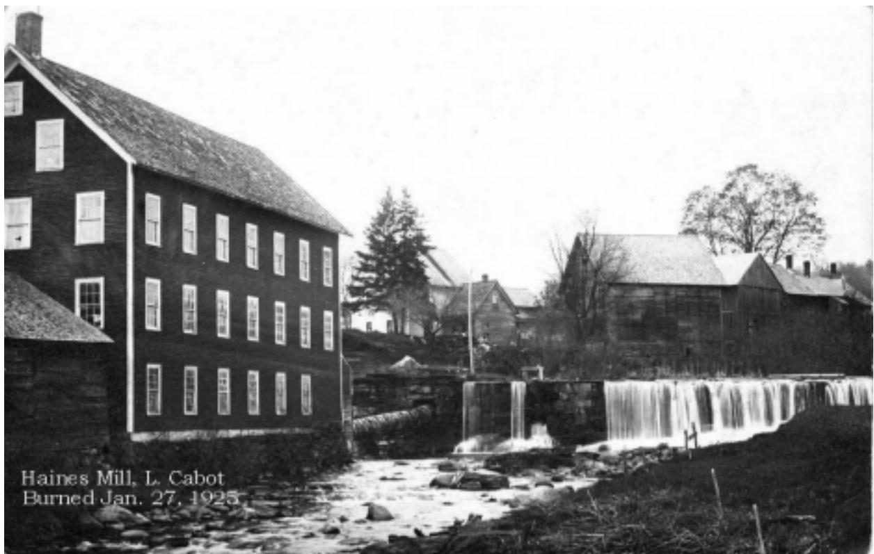
Figure 13. View northwest of the Haines Mill and dam in Lower Cabot (Cabot Historical Society). Note that the dam sluice gate is open (lower left portion of dam).
