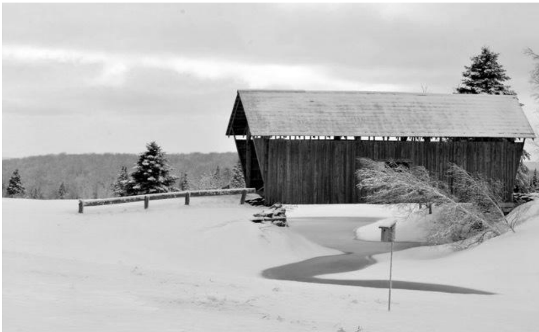
Foster's Covered Bridge, April 2014
