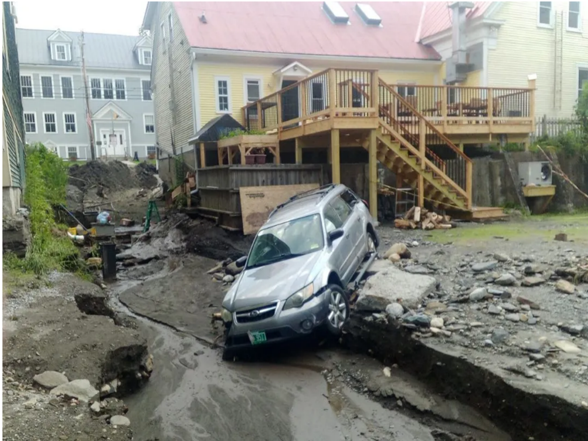
July 2023 Flood Damage
