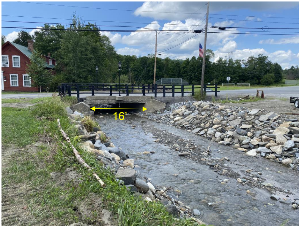
Figure 11: Main Street Bridge viewed from Upstream
