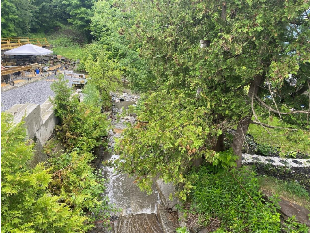
Figure 19: Narrowed Channel Downstream of the Main Street Culverts
