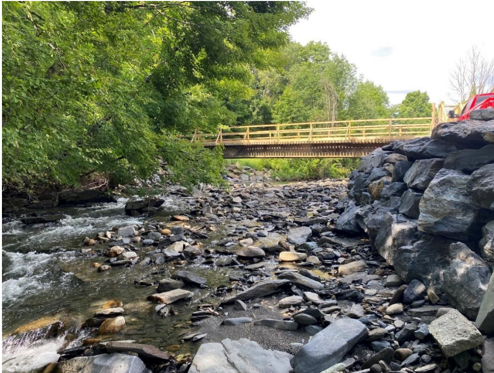
Figure 4: VAST Bridge viewed from Downstream
