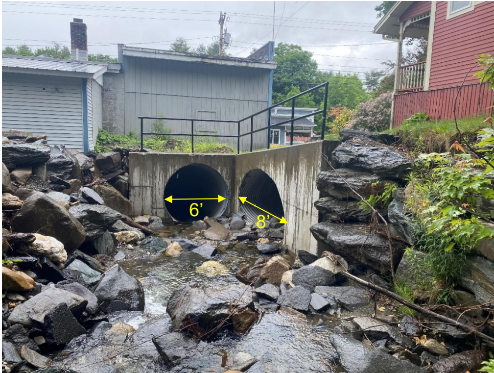
Figure 17: Main Street Culverts viewed from Upstream
