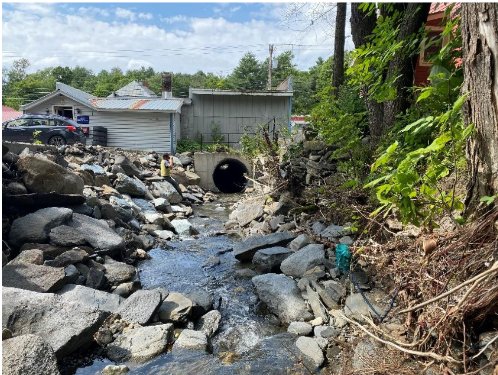
Figure 18: Narrowed Channel Upstream of the Main Street Culverts
