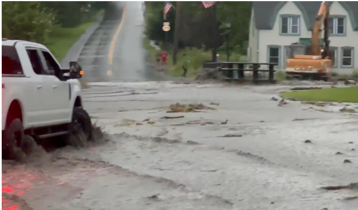
Figure 25: Northern Tributary flood waters overtopping the Main Street Bridge and flowing down Main Street
