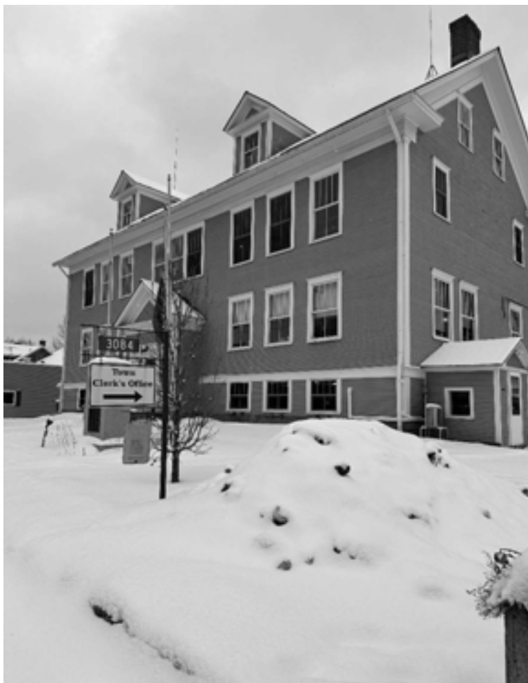
Willey Building, January, 2025 (Picture taken by Brittany Butler)
