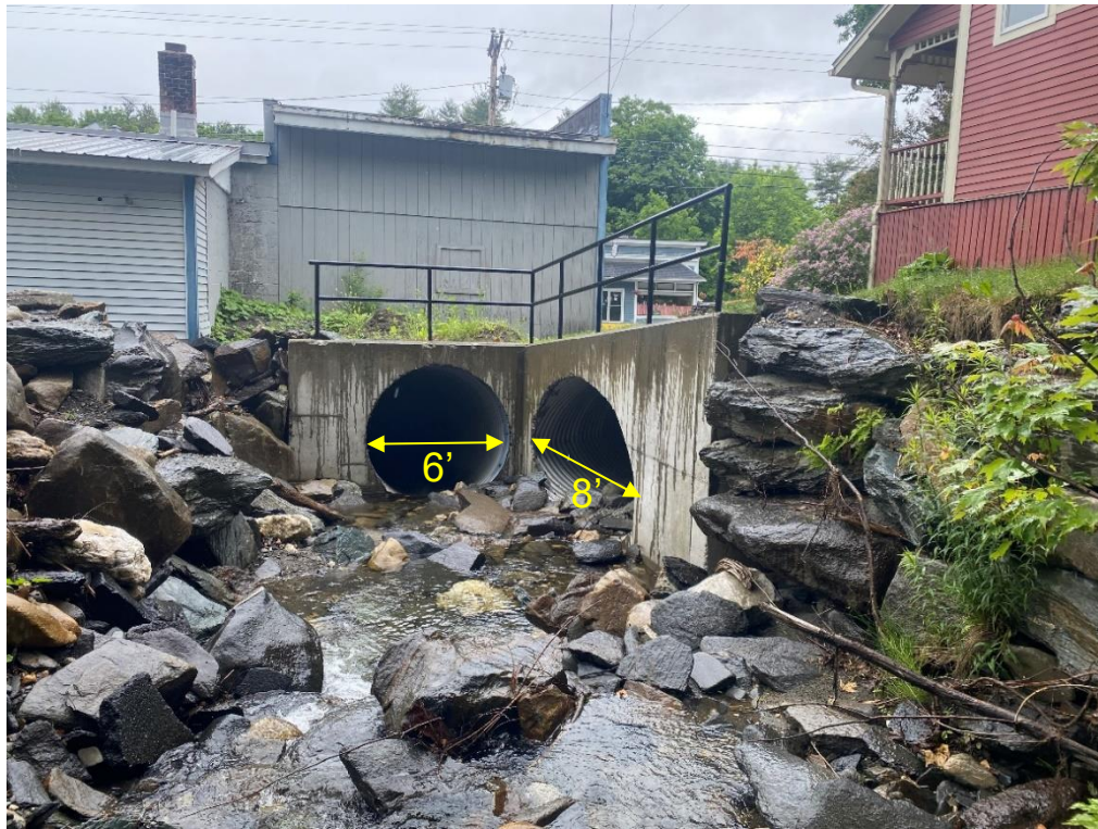
Figure 17: Main Street Culverts viewed from Upstream
