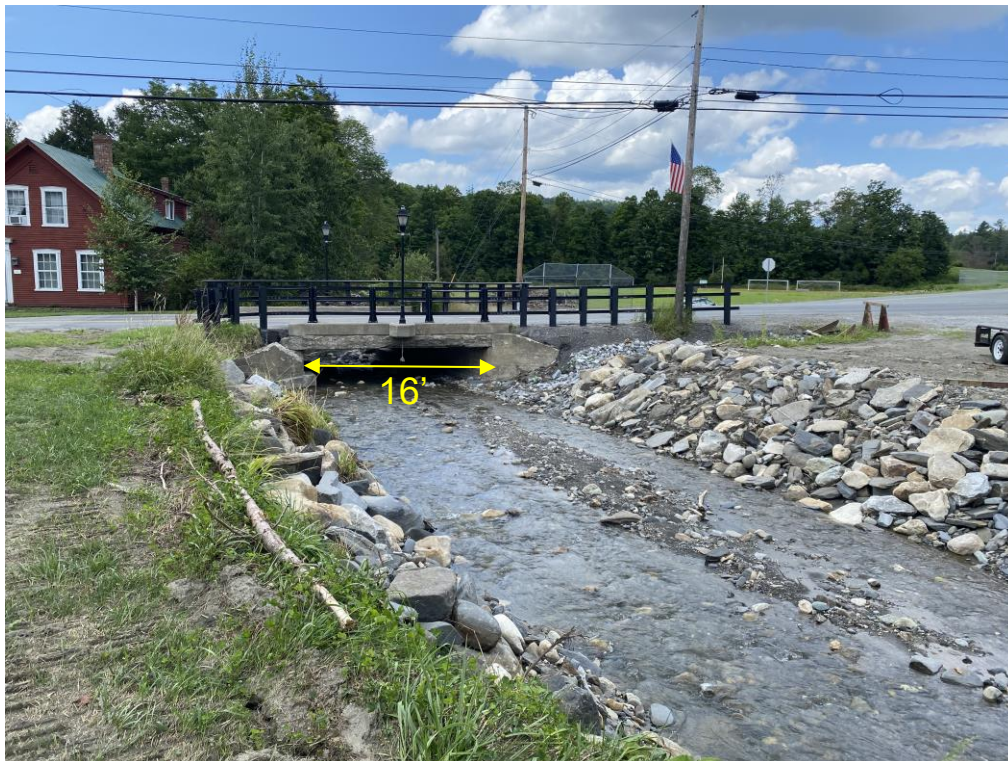
Figure 11: Main Street Bridge viewed from Upstream
