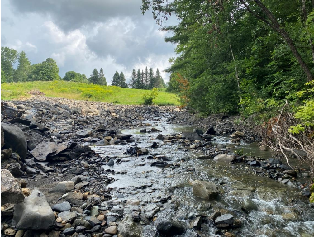
Figure 6: Northern Tributary in Over-Wide Area Post Dredging
